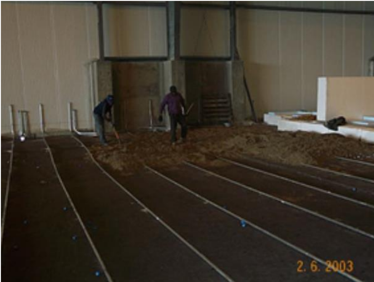
Electric Underfloor Heating System Being Installed
