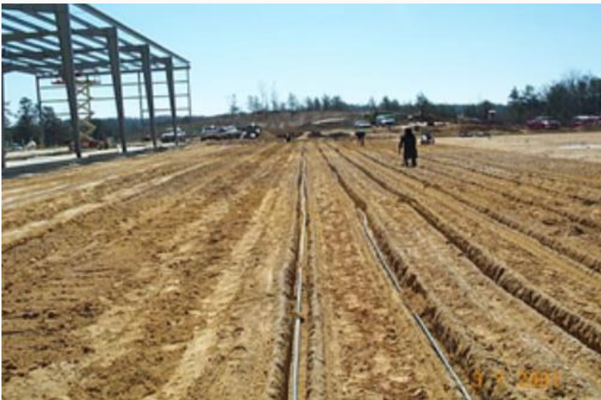
Glycol Tubes Being Laid
