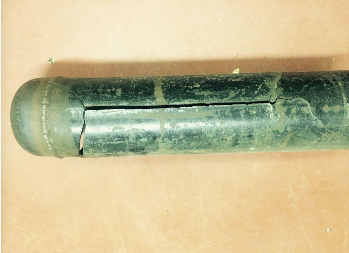
The result of Critical Gas Flow in an Ammonia Refrigeration System
